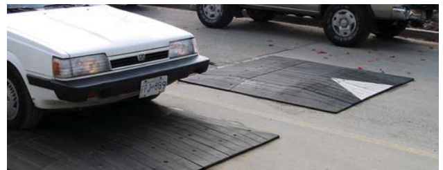
Temporary Speed Cushion
