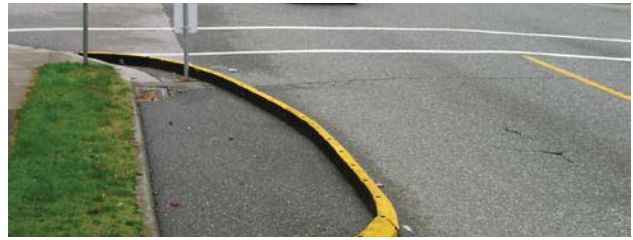
Temporary Curb Extension
