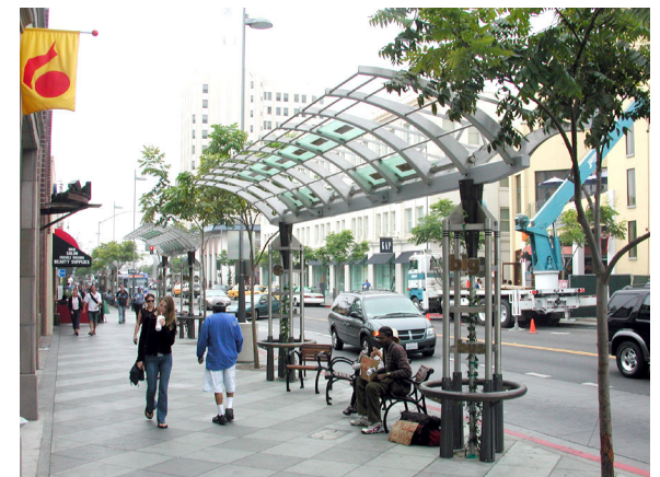
Figure 3-2. Bus shelter in Santa Monica that provides amenities for riders while maintaining the visibility of adjacent businesses.
