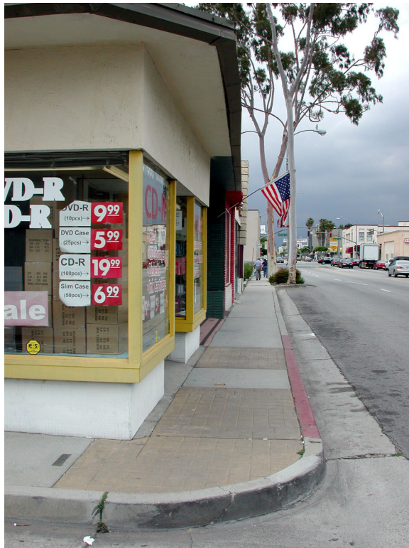
Figure 2-13. Narrow sidewalk on Garfield.
