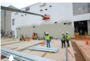
The Multiplier Effect: Data centers provide sustainable job growth BY MARK TONER
