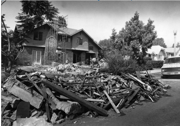
Photo: Whittier Narrows Earthquake Damage 1987 (Source: General Plan - Safety Element)
