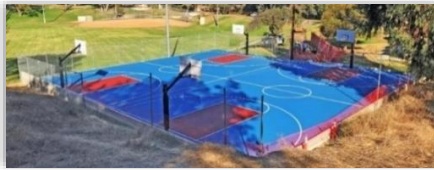
Garvey Ranch Basketball Court Improvements ($500K): This project included construction of new PCC basketball court installation, striping, basketball hoops, fence, and PCC walkway in Monterey Park.
