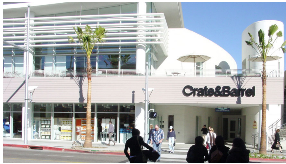
A6. Materials and colors selected to unify the building appearance.
