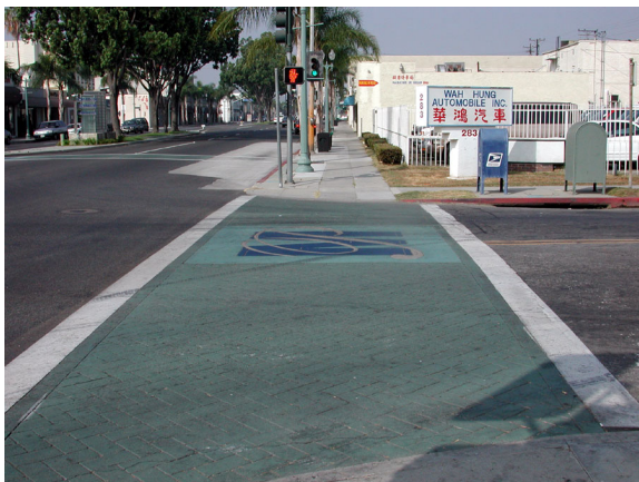
Figure 4-26. Existing decorative crosswalk on Garvey Avenue.
