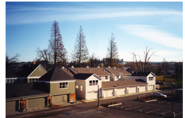
G2. This garage access from an alley includes variation in color, variation in massing, landscaping in setbacks, and a passageway through to live-work units.
