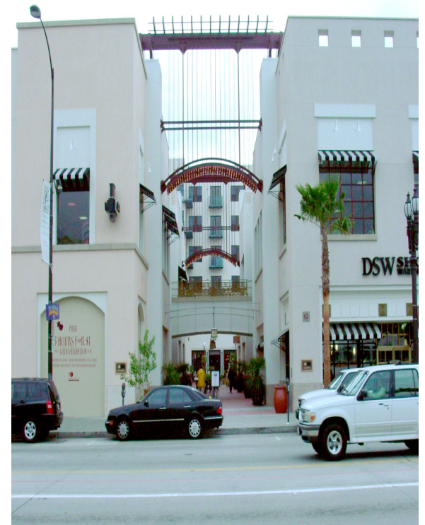
D4. Passageways provide opportunities for light and air.
