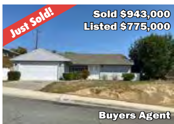
1490 Rockhaven St. Monterey Park
